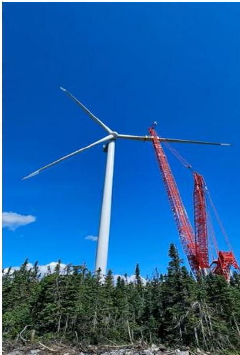
Installation of a turbine at Apuiat wind farm
