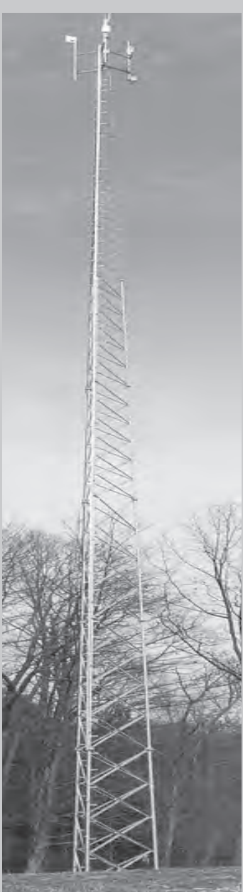
At last, the sky is the limit for Port Ryerse. This photo by Heather Walters was taken late Saturday afternoon, March 10 just west of Port Ryerse on Fletcher's Farm. Kwic Internet had just finished raising the last section of tower into place, and told The Maple Leaf that hi-speed internet will be up and running in about three weeks. Port Ryerse has been one of the more difficult areas to service due to its particular topography, but it would seem that Kwic has finally found the perfect location to provide hi-speed to nearly every resident in that community.
